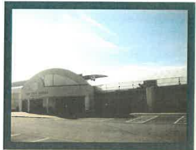
The photo above shows the new Ice Arena Roof.
