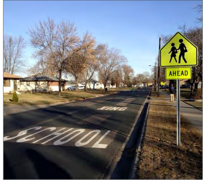
An existing advance school crossing assembly on Unity Ave near Fair Oaks Elementary.
