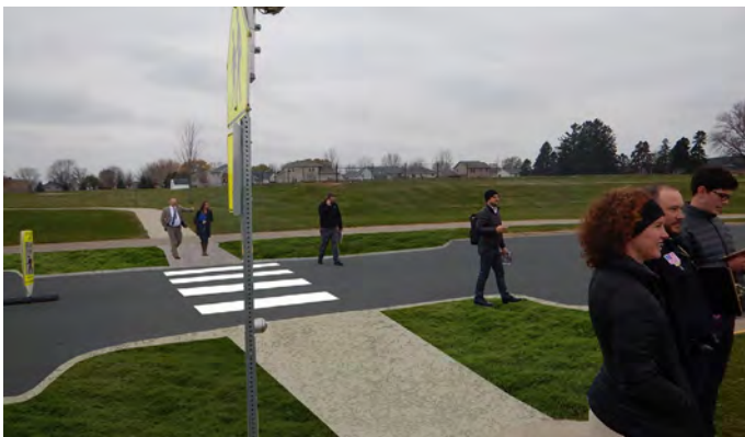
Recommendation I. Midblock crossing of 5th Ave NE between Elementary and Middle School. Curb extensions will increase visibility of pedestrians and help to calm traffic.
