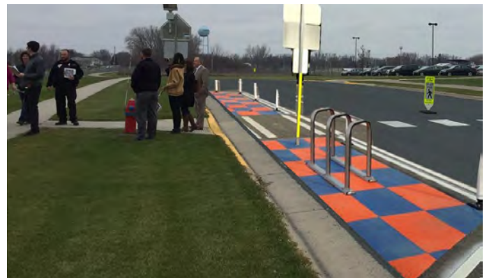
Recommendation I- Alternate. Midblock crossing of 5th Ave between Elementary and Middle School. Example of painted curb extension. This treatment has lower capital costs than a permanent curb extension pictured on the left. It provides protection and increased visibility to pedestrians.
