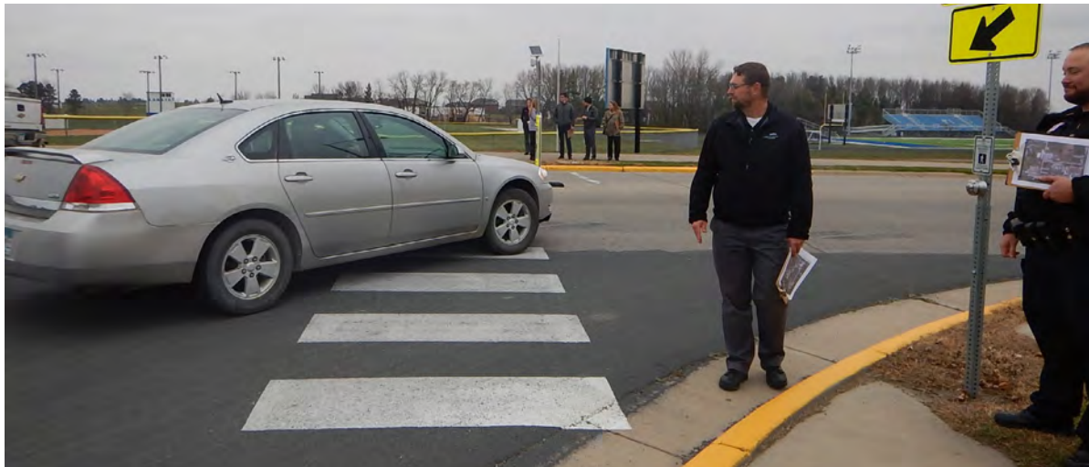
View of 16th St NE crossing at 5th Ave NE. While the crosswalk is marked and signed, the crossing distance is large and vehicle speeds are often high.
