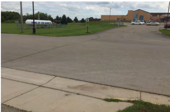
View of 16th St NE crossing from Community Education to parking lot on north side. Notice the wide driveway and lack of separated pedestrian space on south side.
