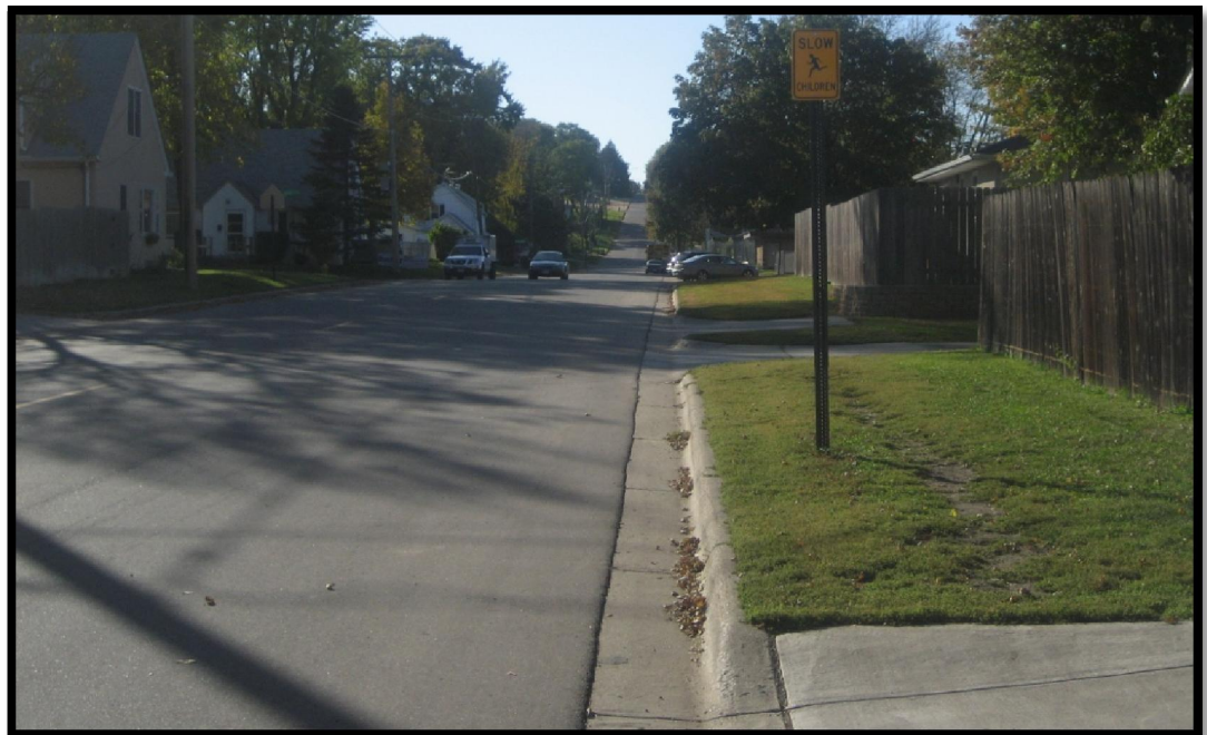
Sidewalk gap on 3 rd Street N between 13 th Avenue and 14 th Avenue. Pedestrian traffic in this block is apparent from the worn path in the grass.
