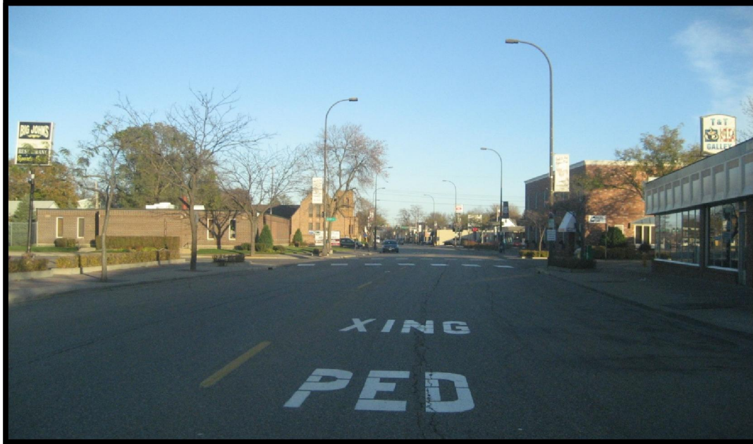
Pavement message and marked crosswalks at the Southview Boulevard/9 th Avenue intersection.
