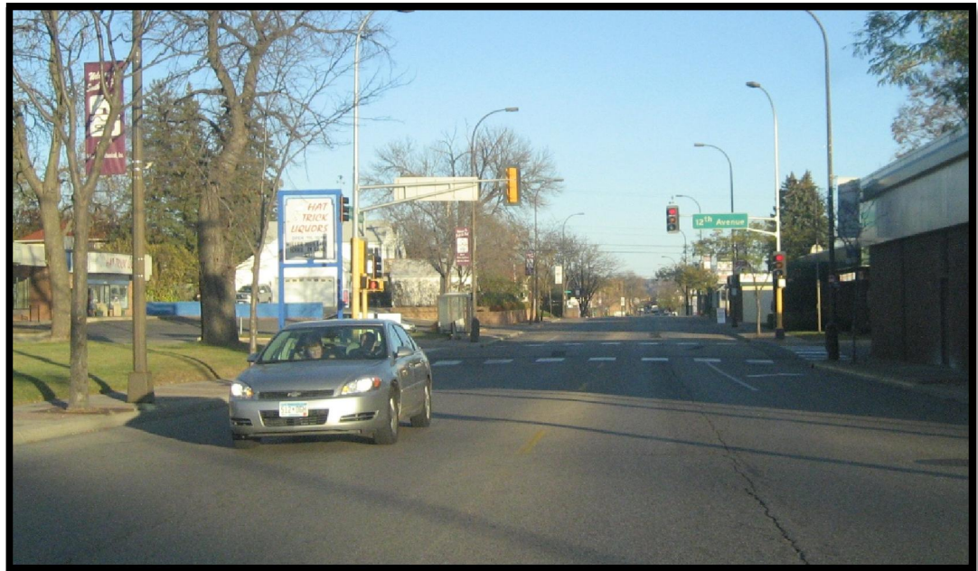
Existing conditions at the Southview Boulevard/12 th Avenue intersection.
