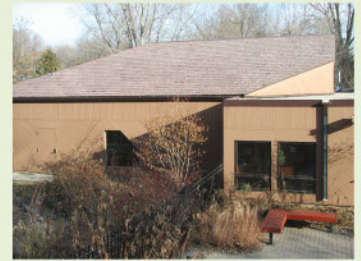
Finished Eco-Shake Roof
