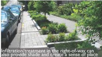
Infiltration/treatment in the right-of-way can also provide shade and create a sense of place
