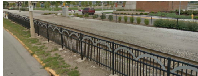
Decorative railings and plantings provide a barrier between railroad right of way and vehicular and pedestrian spaces.
