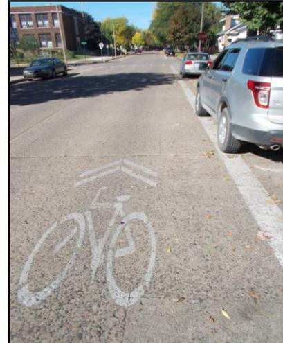
Following the completion of the SRTS work, the City of Lewiston will fund and direct the Public Works Department to paint sharrow markings on Williams Street an estimated 2,640 feet; County 25 from Highway 14 to the south city limits an estimated 5,280 feet; Fremont Street from Highway 14 south and continuing on County 29 south to the city limits an estimated 5,280 feet.
