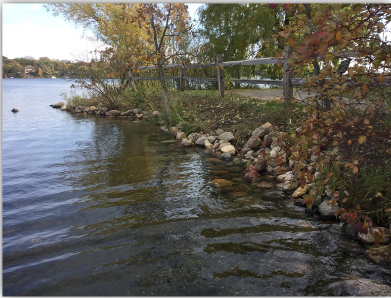
(Above) Rocks were hand placed on the Lake Marion shoreline in areas where wave action causes high erosion.
