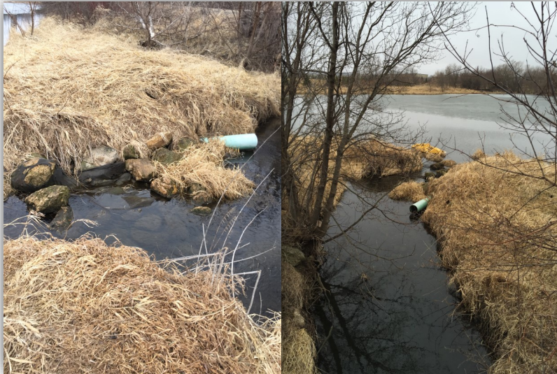
(Above) Pond outlet prior to restoration.
