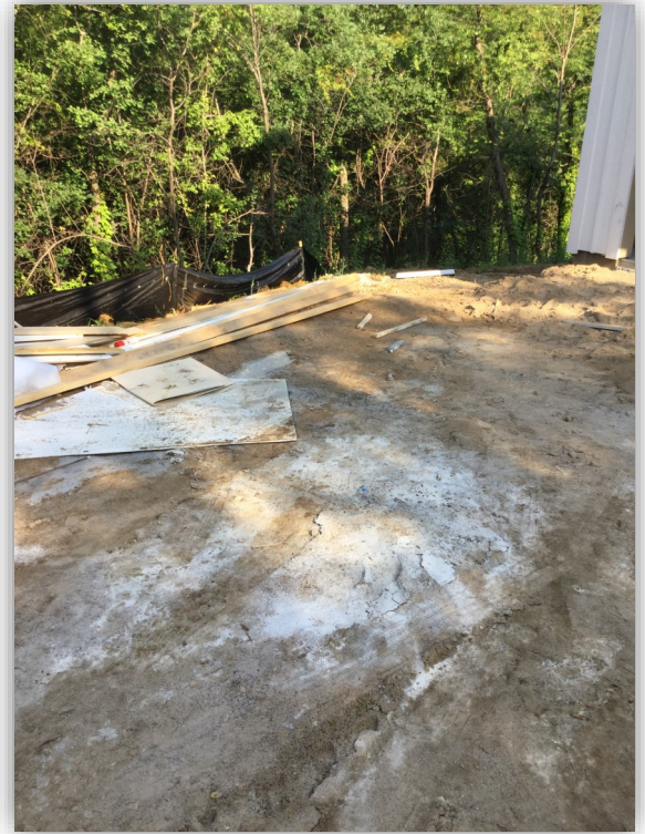
(Above) Concrete washout is toxic to plants, aquatic organisms and contaminates groundwater.
