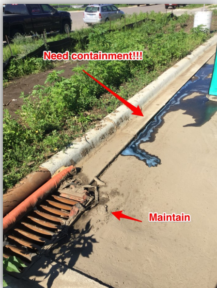
(Left) Secondary containment is required for bathroom facilities—without containment, hazardous waste can enter stormwater infrastructure.
