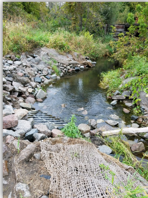
(Above) Pond outlet post construction.
