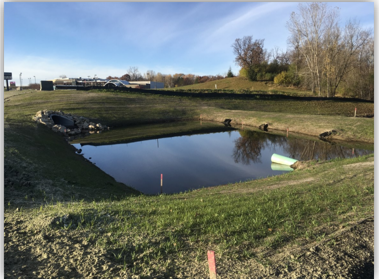
(Above) A temporary bypass was installed during construction to allow for pond vegetative growth.
