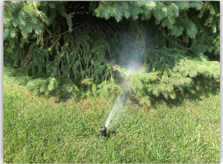
(Above) Sprinkler spraying into a conifer (area not meant for irrigation).
