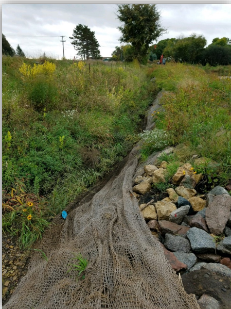
(Above) Native seed post construction.
