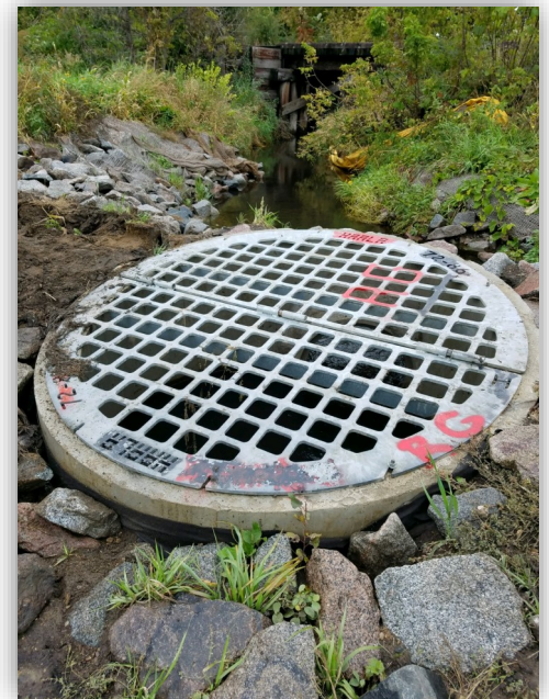
(Above) Emergency overflow structure.
