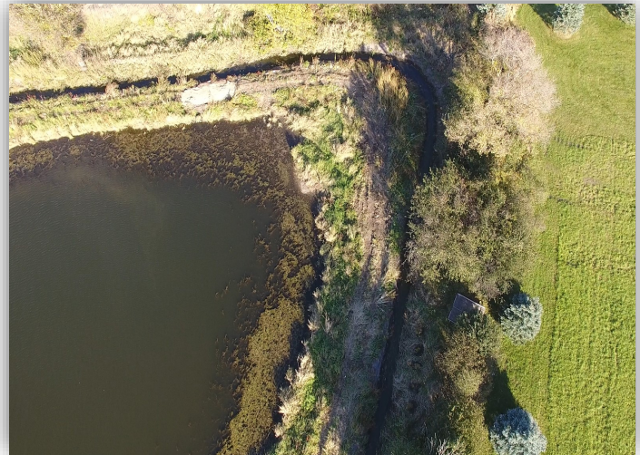
(Above) Stabilized channel post construction.
