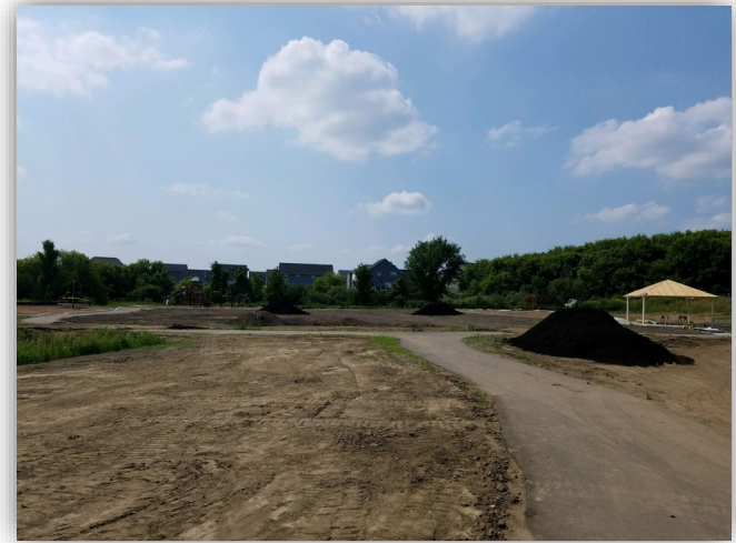
(Above) Compost awaiting spreading during park construction.
