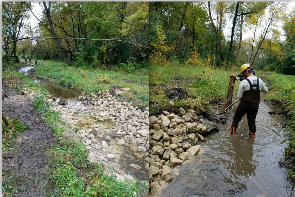
(Above) Rocks and tree stumps created additional stabilization in high channel flow areas using bioengineering.
