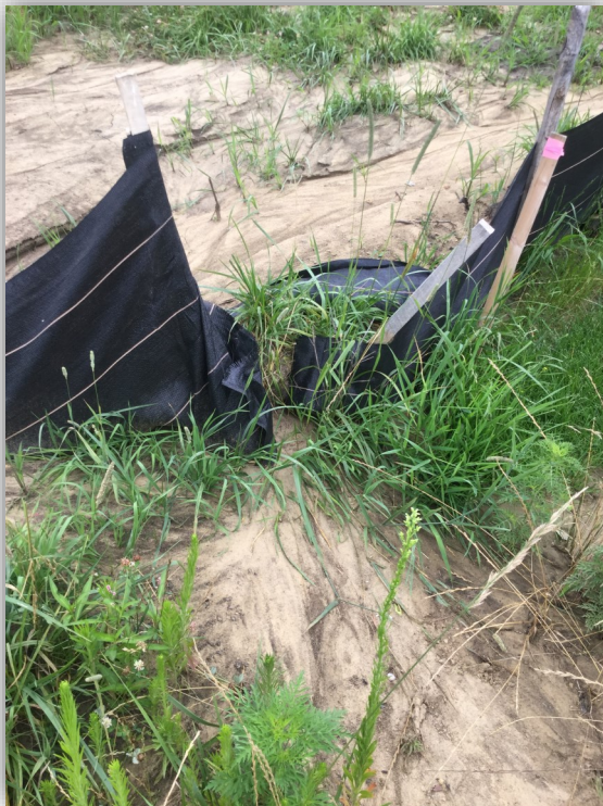
(Left) Silt fence that is not maintained (cleaned once half full) becomes bypassed during heavy rains, which results in sediment deposition on neighboring lots.
