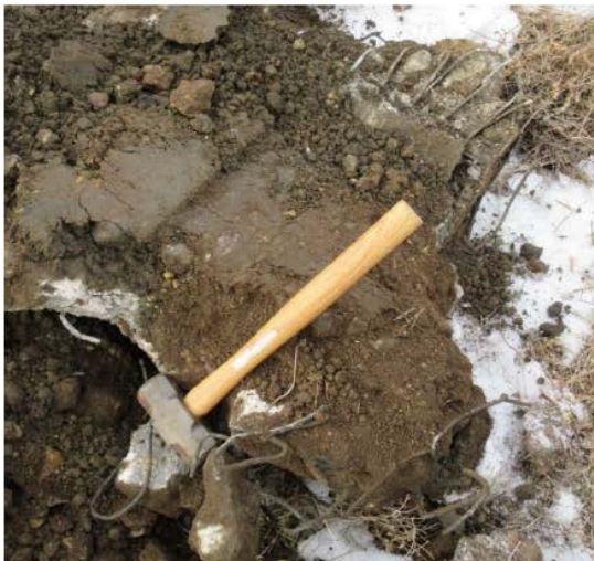
Figure 5. Concrete with rebar observed at TP-7
