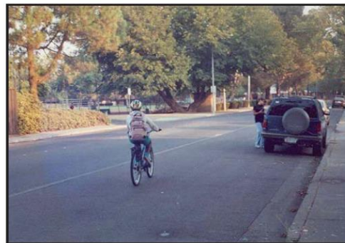
Wide Paved Shoulder
