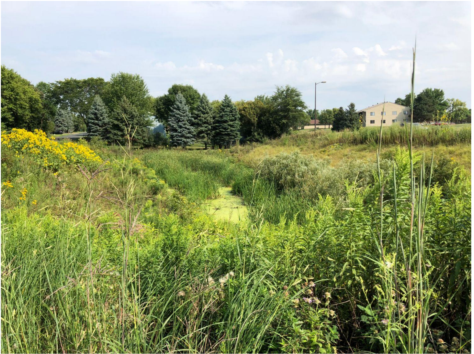
Storm Pond Buffer- Aug. 2018
