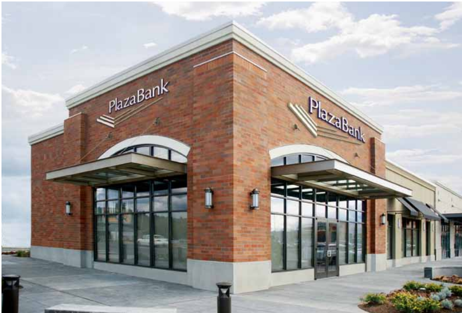
Destination oriented retail and service uses are likely candidates near the intersection of Highway 7 and 15.
