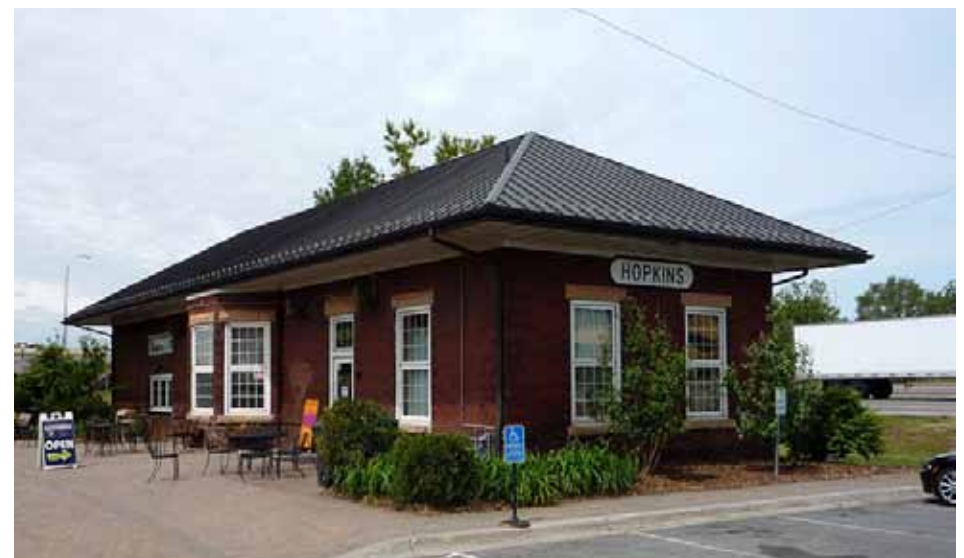
The renovated depot in Hopkins, MN serves as a trailhead and coffee shop
