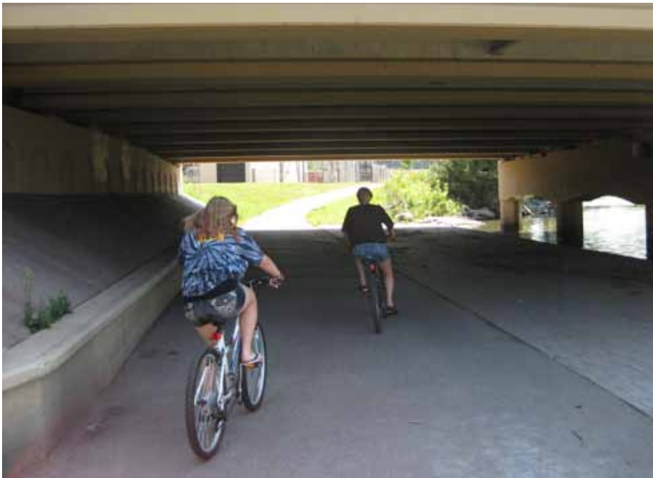
The new grade separated trail crossing of Highway 15 for the Luce Line Trail
