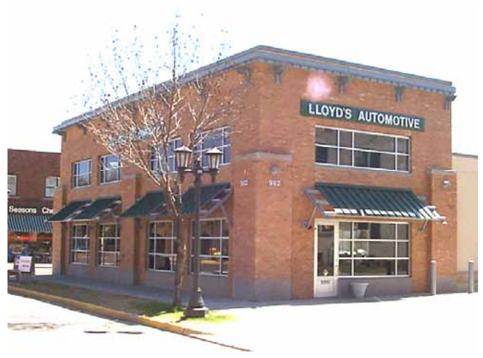
New development projects should respect the size, scale and details of historic architecture down-
