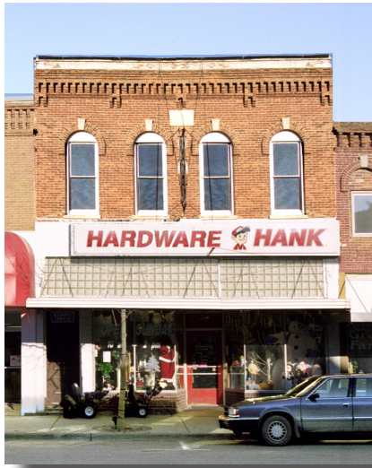
Backlit plastic signs and underlit awnings with lettering are inappropriate for historic buildings.
