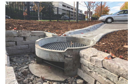
Pretreatment structures filter rainwater runoff
