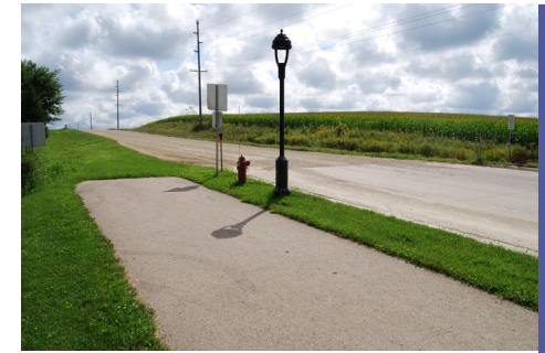
16th St. NE is currently only paved to the edge of the developed portion of Kasson.
