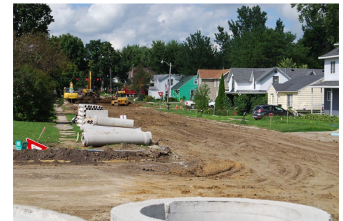
Summer 2017 Kasson Road Reconstruction
