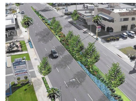
Landscaped medians are some of the most effective means to regulate access and reduce crashes.
