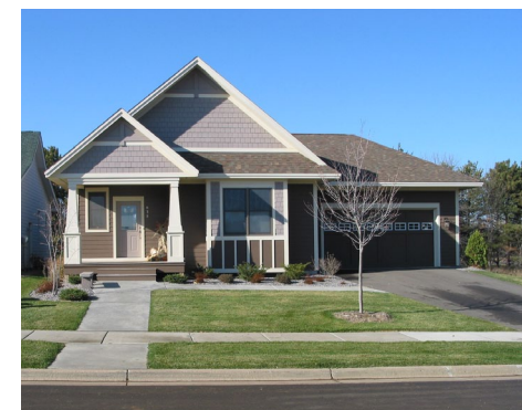
Subdivisions should have sidewalks and homes with design features that minimize the presence of the garage along the street.
