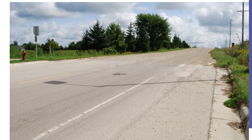
16th Street Transition from Paved to Unpaved
