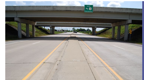
US Hwy. 14 Overpass Over Hwy. 57
