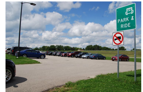
MnDOT Park and Ride Facility
