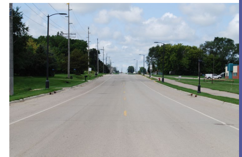
16th St. NE caters to a variety of roadway users.
