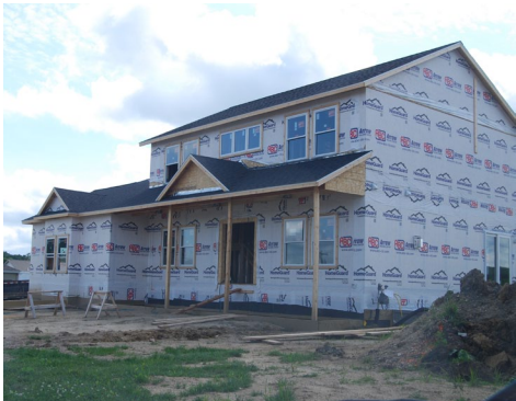
New Home Under Construction in Kasson
