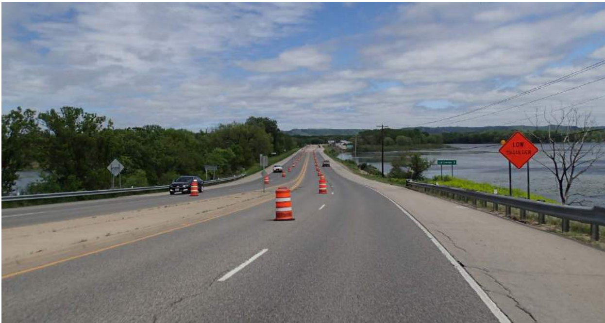
Figure 7. US 14 connection to West Channel Bridge (under construction Summer 2017)
