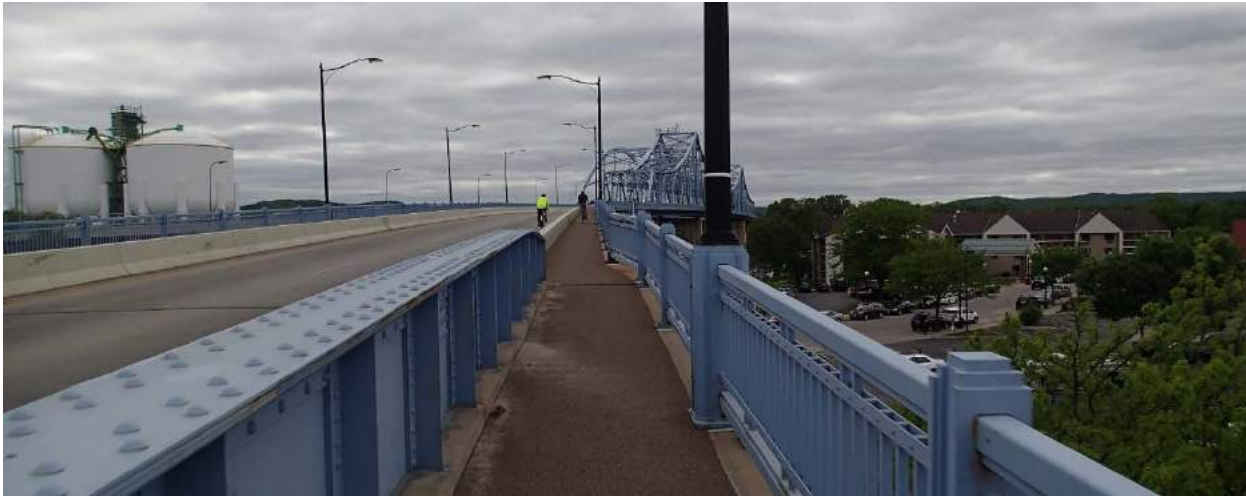
Figure 10. Sidewalk and shoulder on Cameron Avenue Span
