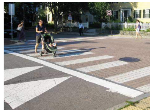
Raised crosswalks are an effective means to calm traffic on lower-volume streets.
