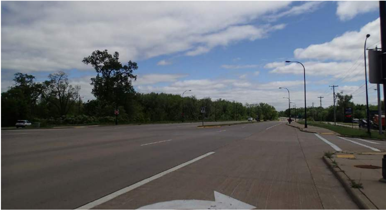
Figure 8. Sidewalk along US 14, with shoulder interrupted by turn lane
