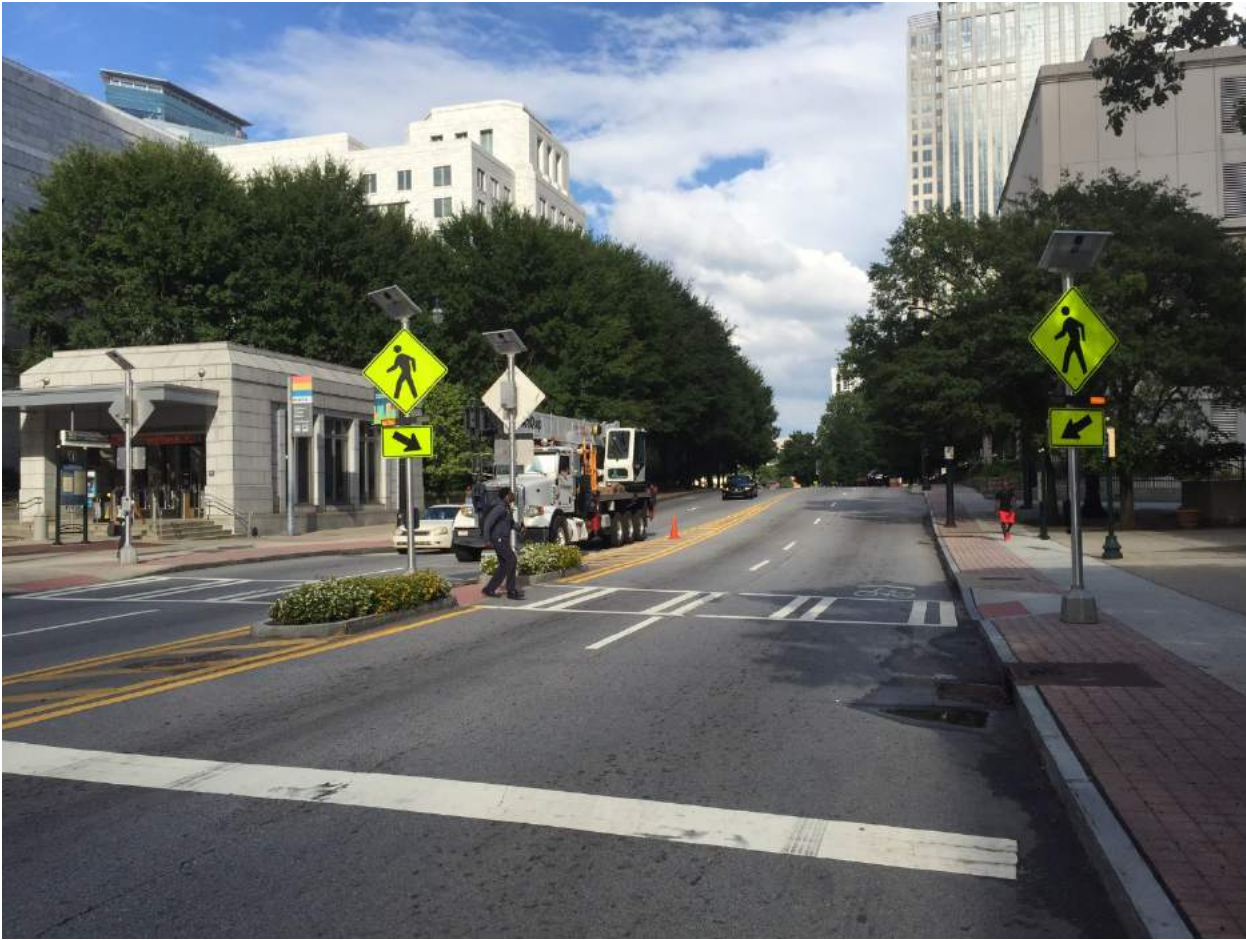
Figure 6. A pedestrian crossing featuring a Rectangular Rapid Flashing Beacon (RRFB). High intensity flashing lights are activated by a pedestrian needing to cross.
