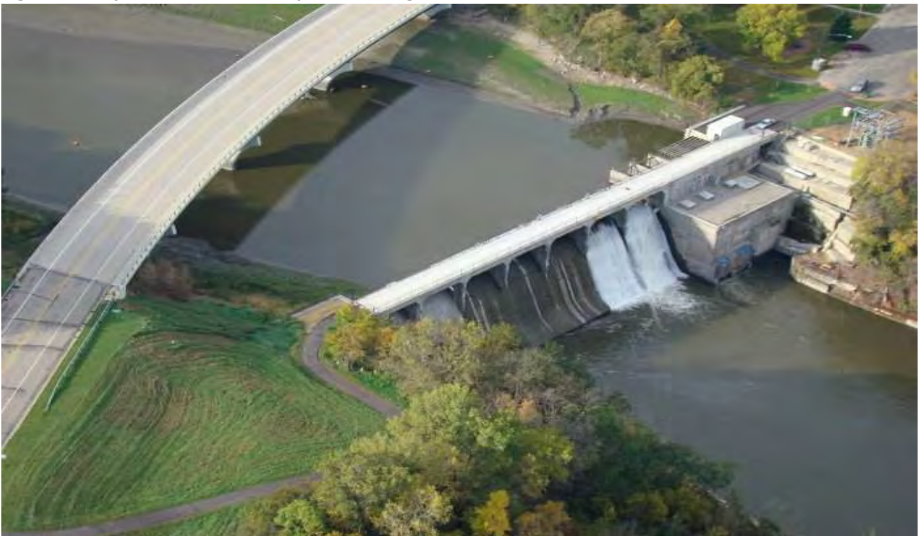
Figure 18: Rapidan Dam and County Road 9 bridge on Blue Earth River.
