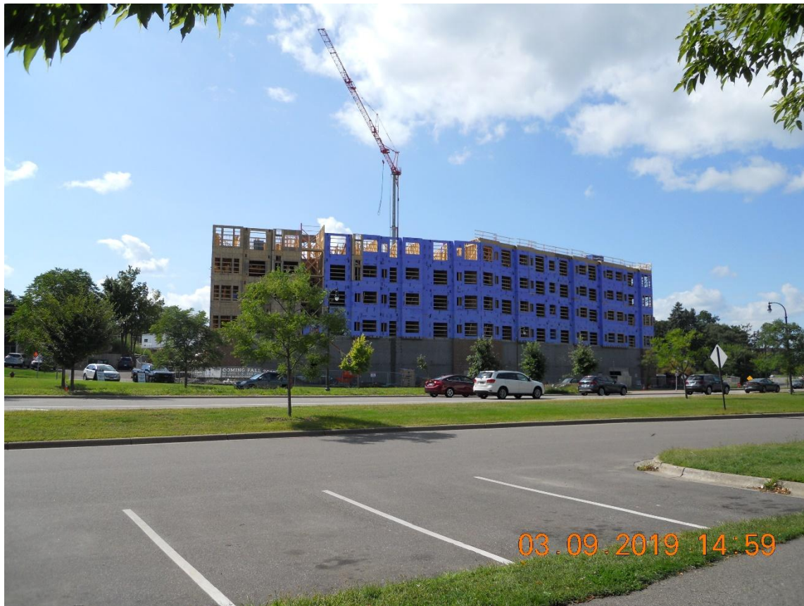
Figure 10: Birdtown Flats Apartments Under Construction
