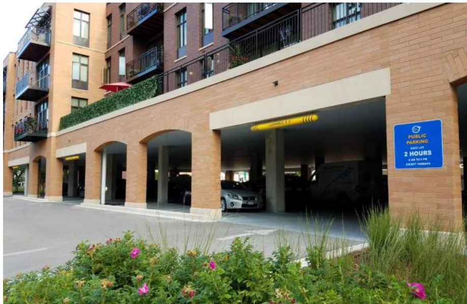
Figure 26. Example of a new construction redevelopment that retained existing surface parking for public use, and built new additional underground spaces for the residential development above.
