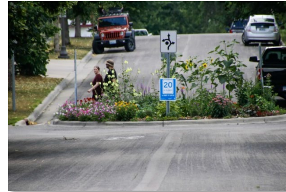
▲ Traffic circles help achieve neighborhood-friendly speeds of 15-20 mph by design. (Saint Paul, MN)
