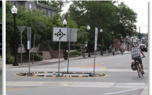
▲ Traffic circles can be tested using low-cost materials. They keep people safely in motion, which is beneficial to people biking. (Edgewater, CO)
