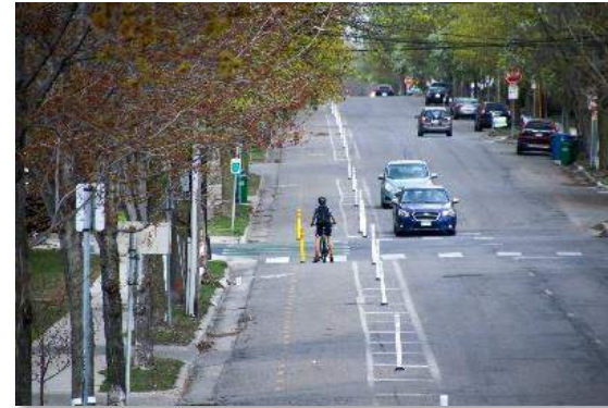
▲ Two-way protected bike lane using a painted buffer space and flex posts to create vertical separation. (Minneapolis, MN)
