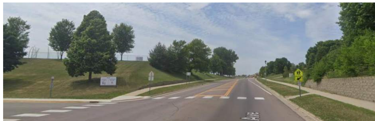
There are two marked and signed crosswalks near the middle school; however, they lack any type of beacons or median crossing island to enhance visibility. Photo Source: Google Streetview.
