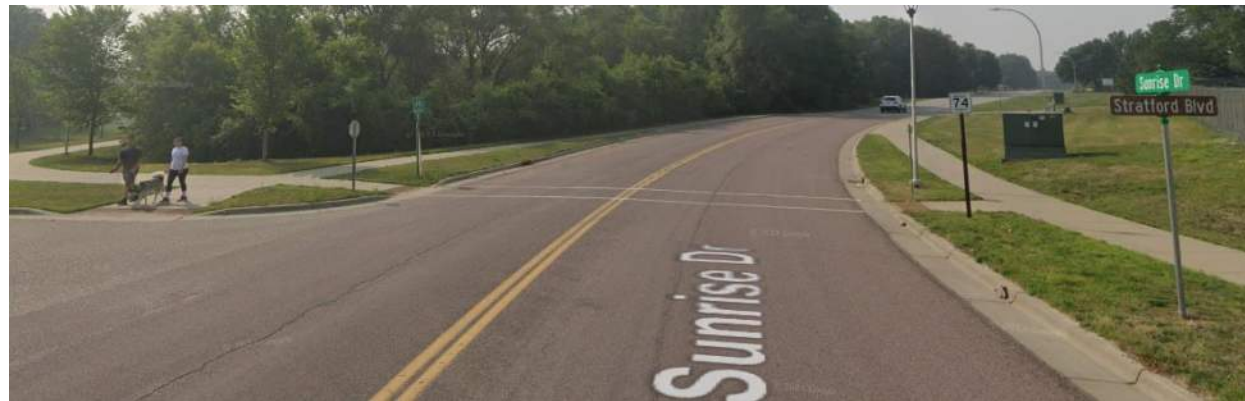
Pedestrians walk along Sunrise Drive. The marked crosswalk lacks crosswalk signage and high visibility markings. Photo Source: Google Streetview.
