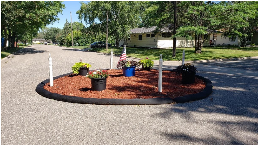
A traffic circle can be used as a traffic calming device in high-traffic areas. Photo courtesy of Tim Schoonhoven.
