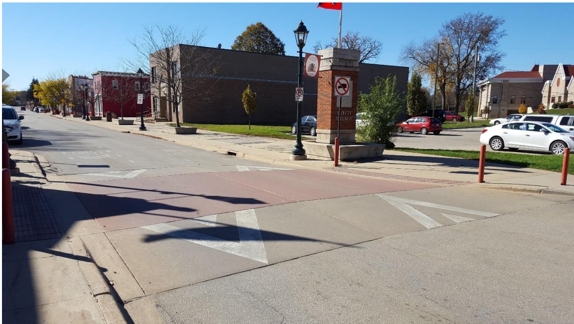
Speed tables, or raised crosswalks, are midblock gradual speed bumps that also function as a crosswalk for bicyclists and pedestrians. They help calm traffic speeds and provide more awareness for pedestrians and bicyclists crossing. Image courtesy www.pedbikeimages.org / Brandon Whyte.
