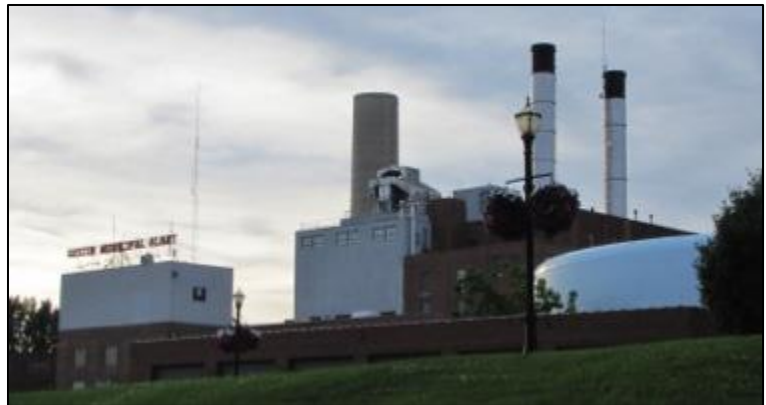
Austin Municipal Power Plant Photo Credit: CR Planning
