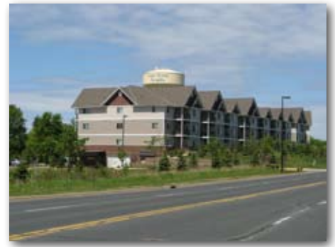
Inver Grove Heights Water Tower
