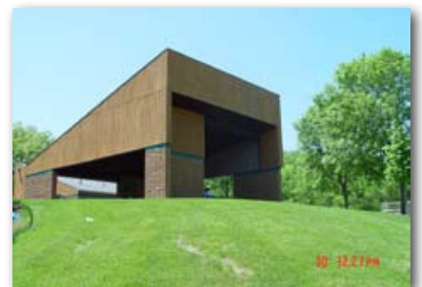
South Valley Shelter
