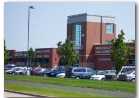
Eagan Transit Center with retail development adjacent a park and ride lot. Retail parking demands generally have opposite peak demand than commuter parking and therefore creates opportunities for shared parking.
