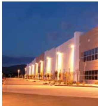
Exterior lighting should use full cut-off fixtures that prevent light trespass and glare, especially as seen from the marsh
