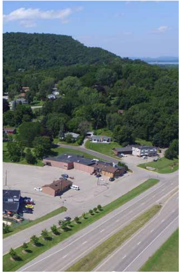
The American Legion site on North Chestnut St. offers excellent exposure and access to the highway for a new use such as a hotel.
