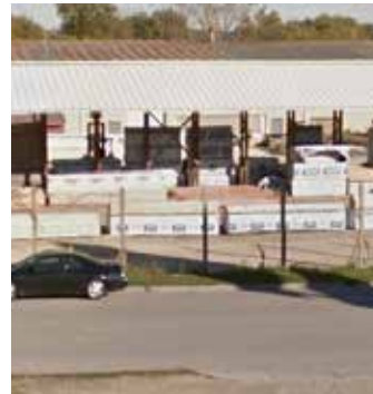
Storage and loading areas should be screened from view from the highways
