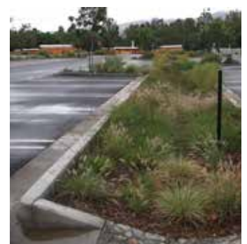
Parking lot landscape islands can also collect and filter stormwater runoff
