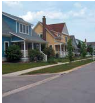
Narrow lots and shallow front yard setbacks are encouraged, to use land efficiently
