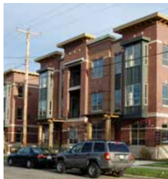
Larger buildings should use various strategies to minimize apparent size, including projections, varied rooflines, etc.
