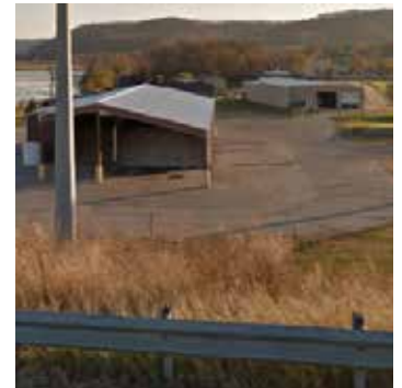
Buildings that are lower than the adjacent highways should not have rooftop mechanical equipment
