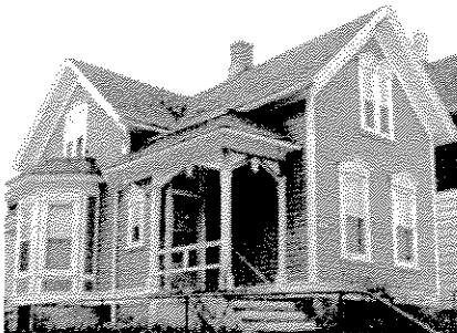
Victorian: The steep roof, porch and high windows are dominant.
